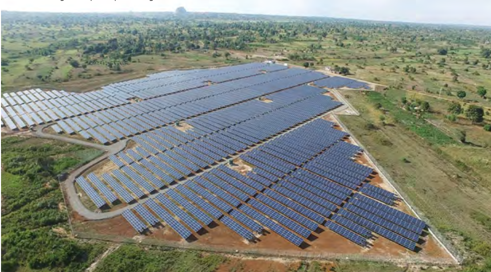
East Africa's largest PV power plant in Uganda
